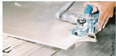
After demounting tapers can be easily reformed making reuse possible.
